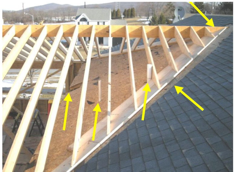
The installation of flashing in the new valley is shown. Note that existing shingles have been removed and ice and water barrier has been applied.
